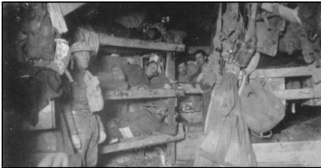
Example of a sleeping dugout built and used by the Australian Tunnelling Companies, WW1.
