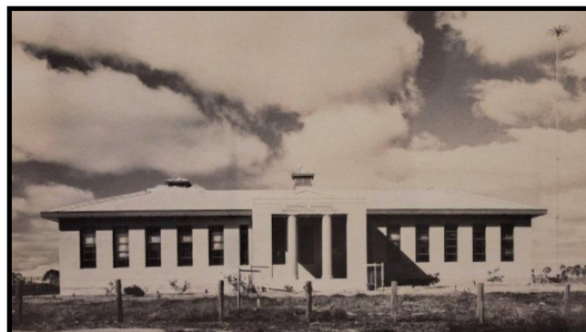
2CR Station & Antenna, Cumnock, 1939.
